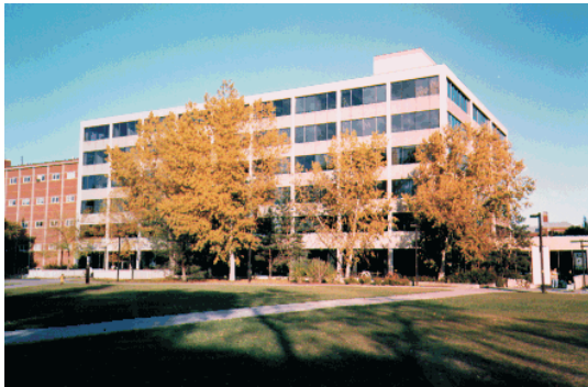
Central Academic Building, PIMS-UA Site Office
