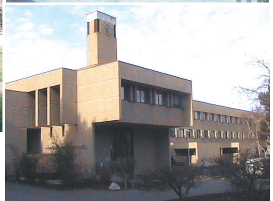
Clearihue Building, UVic Site Office
