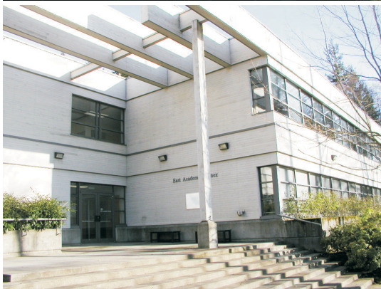
East Academic Annex, PIMS-SFU Site Office
