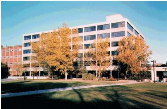
Central Academic Building, PIMS-UA Site Office
