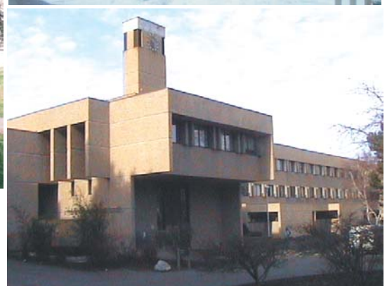
Clearihue Building, UVic Site Office
