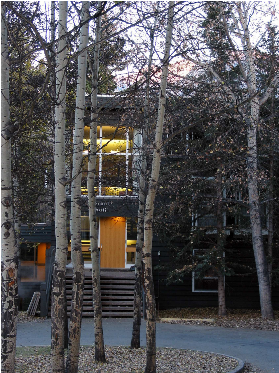
Corbett Hall at the Banff Centre on a fall morning.
